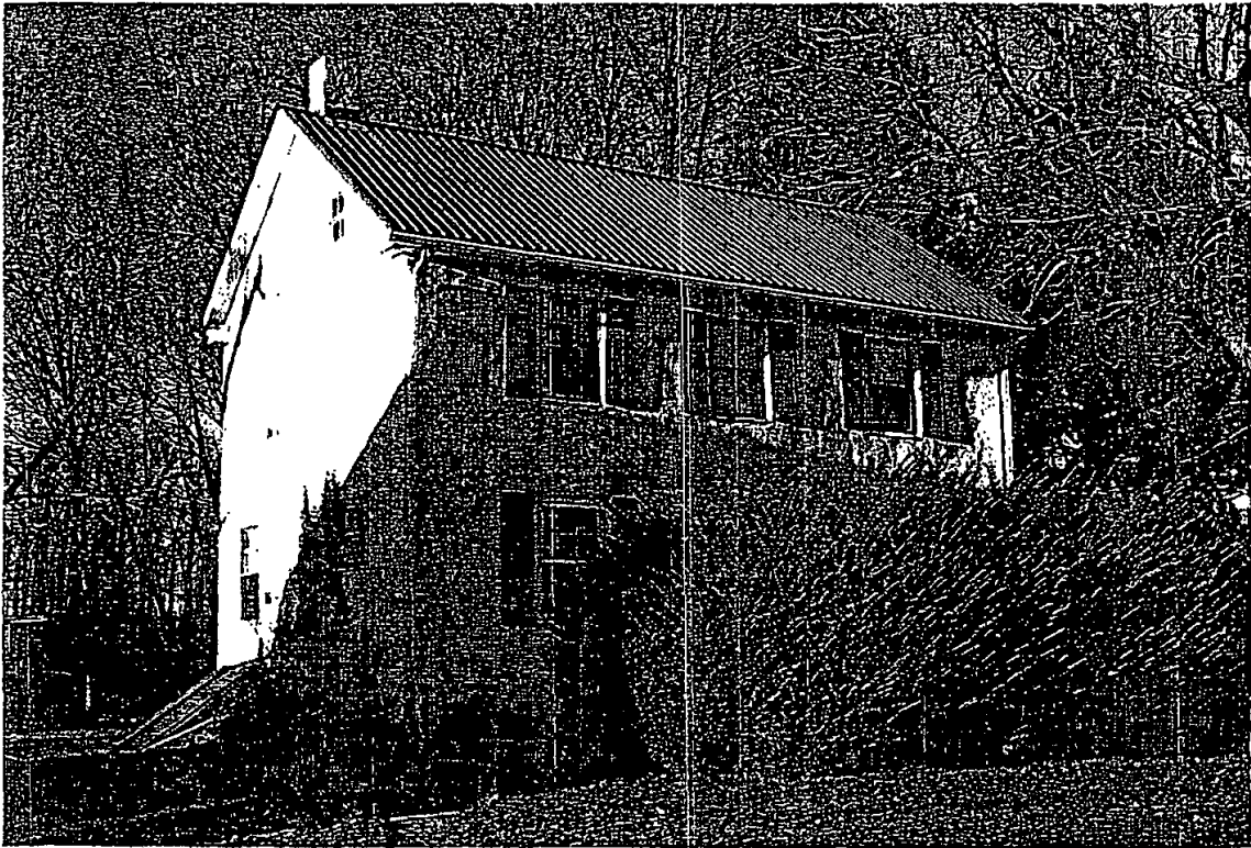
South elevation of house.
