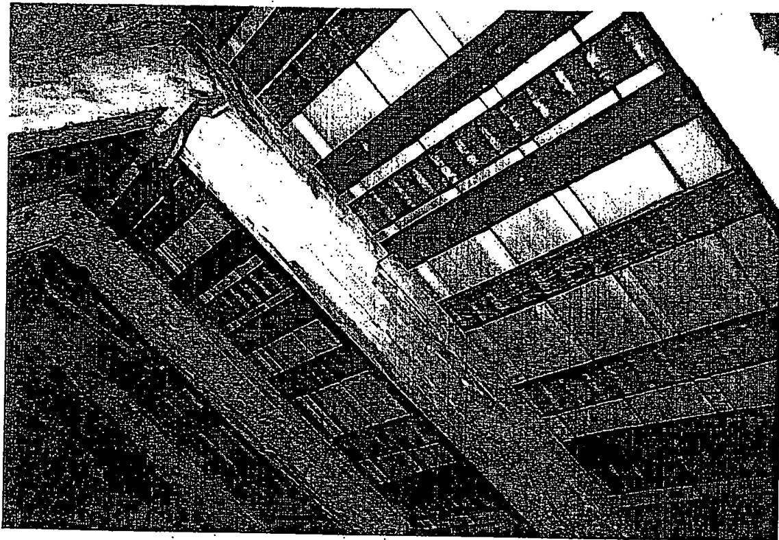
Exposed roof framing in attic of main house.
