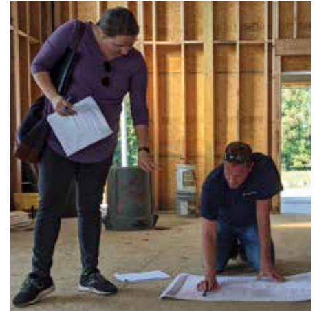
Bottom: Jester Artspace Construction Chair, Suzanne Murphy discusses interior fit out with Brian Smith of BSS Contractors, October 21, 2021.
